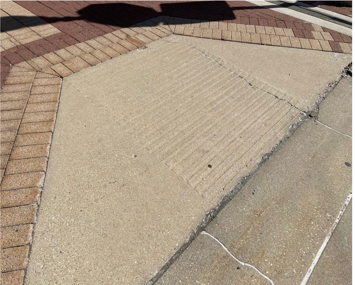
ADA Warning Exp.-Alert texture in pavement, Prairie Park
