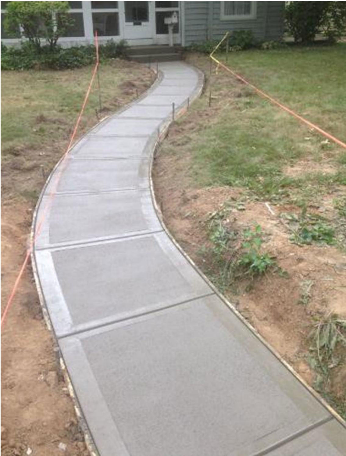
All Sites - Exp of concrete finish
