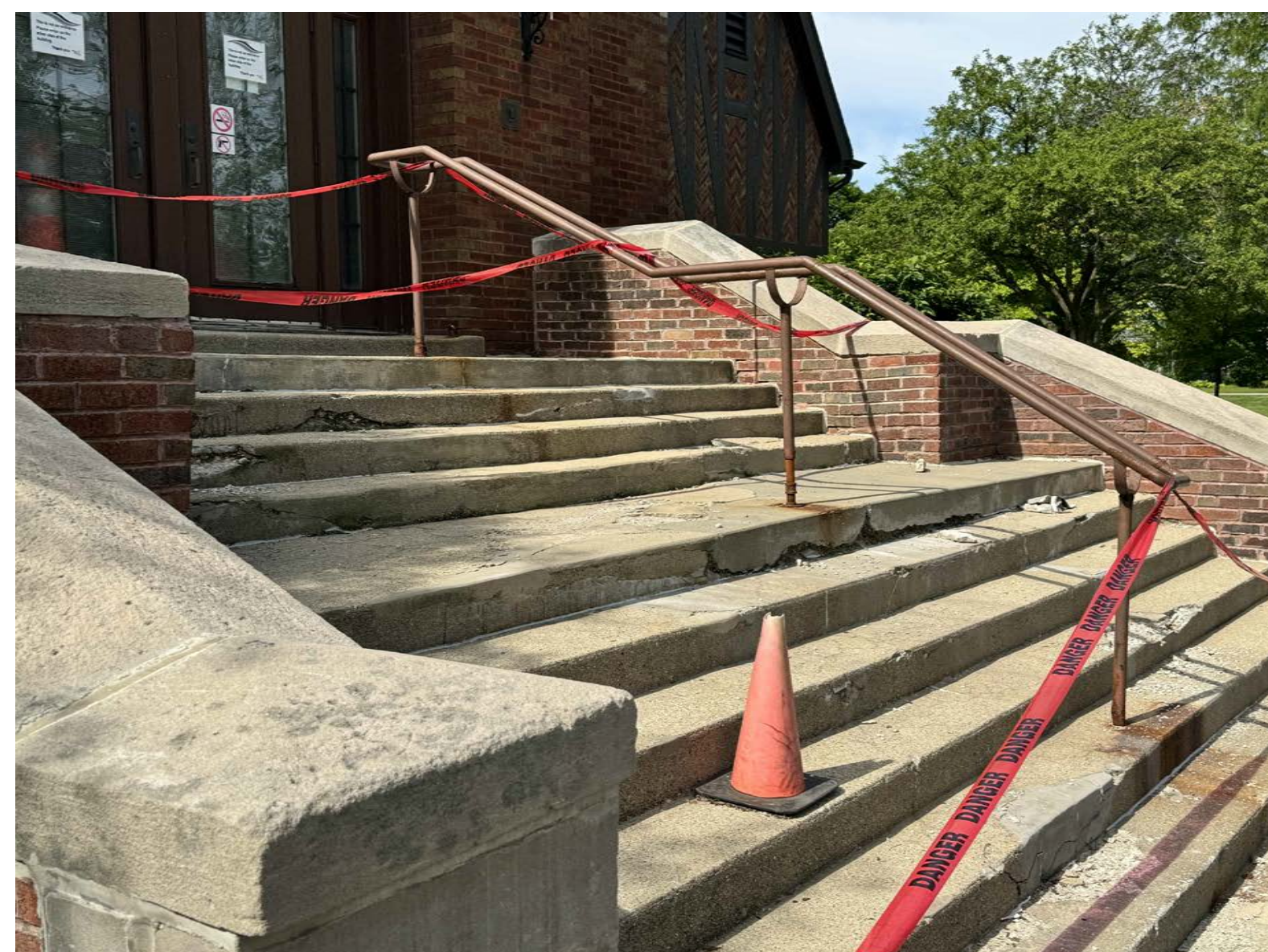
NORTHEAST SIDE OF STAIRS - ZOOM
