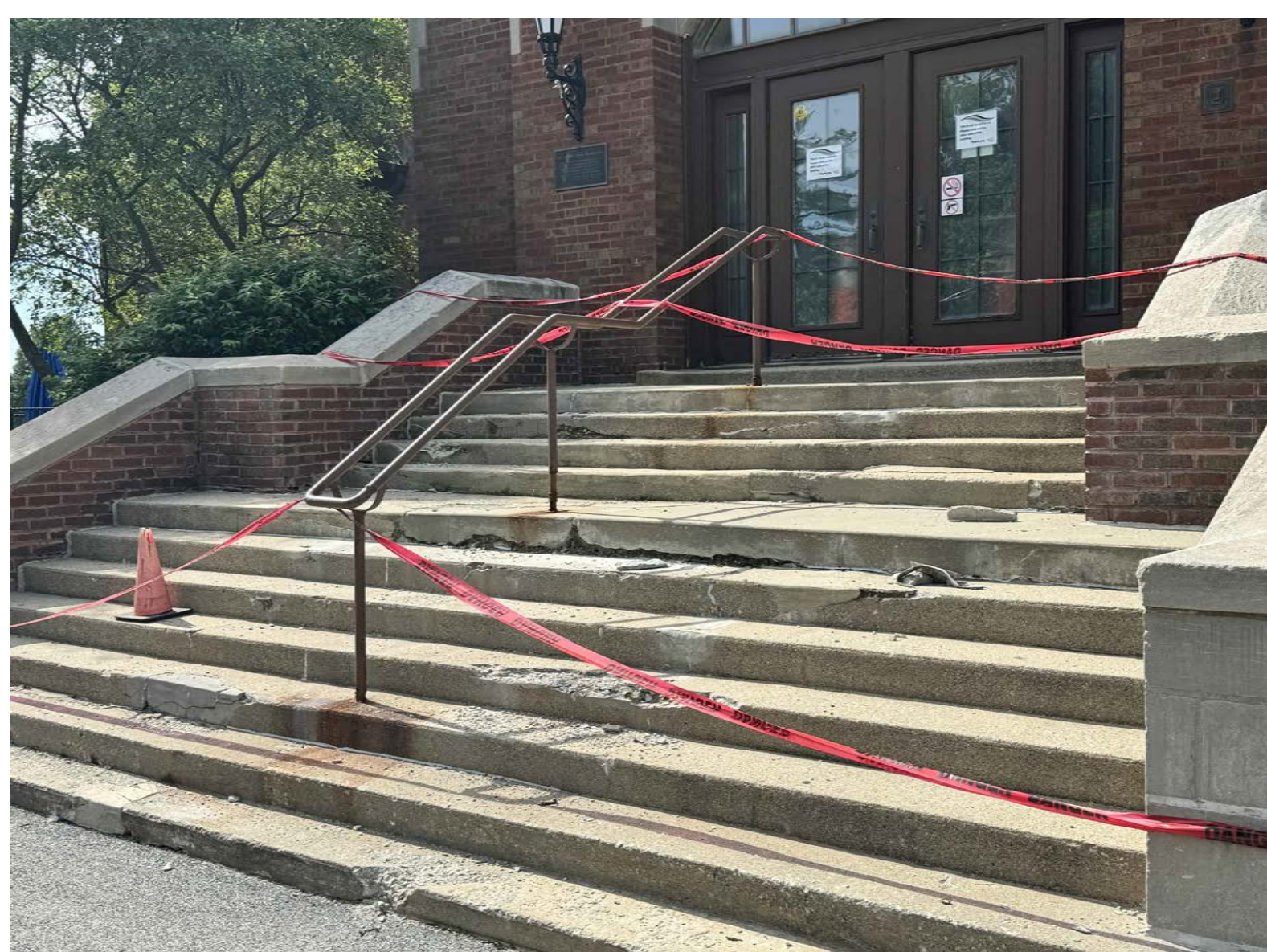
NORTHWEST SIDE OF STAIRS - FULL VIEW
