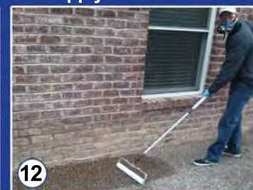
Apply Roller Coat
